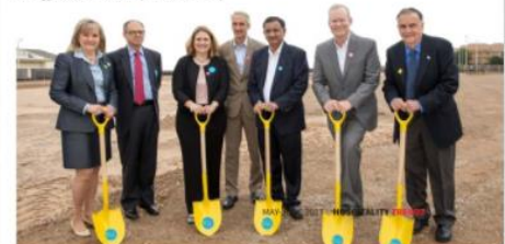
Breaking ground on the first ever Tru by Hilton in Oklahoma City.
